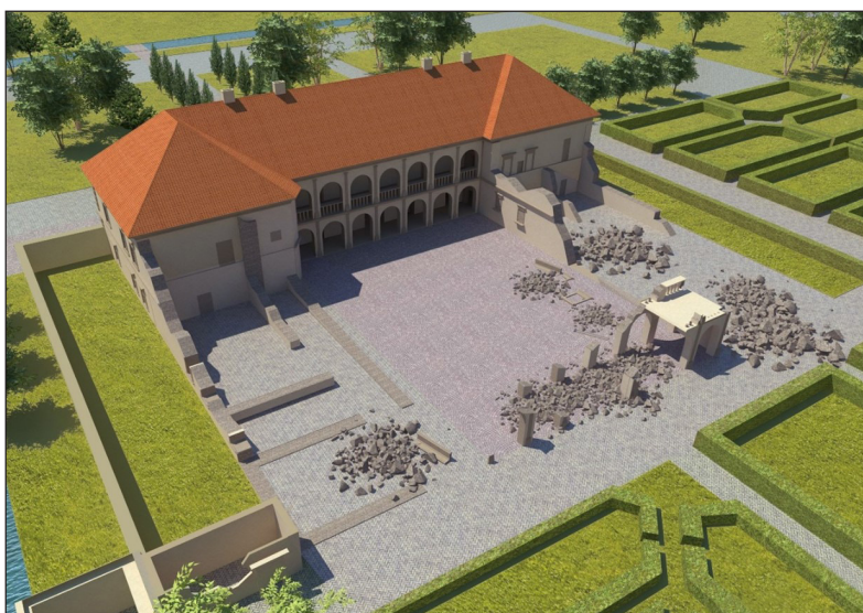
Figure 9: The Łobzów palace after its reconstruction by John III Sobieski, digital reconstruction of the probable state of the building's preservation from the final decade of the seventeenth century, after the gradual demolition of the remains of the eastern, western and the entirety of the northern wing so as to obtain materials that could be used in the construction of the Palace in Wilanów; author: Piotr Pikulski.
