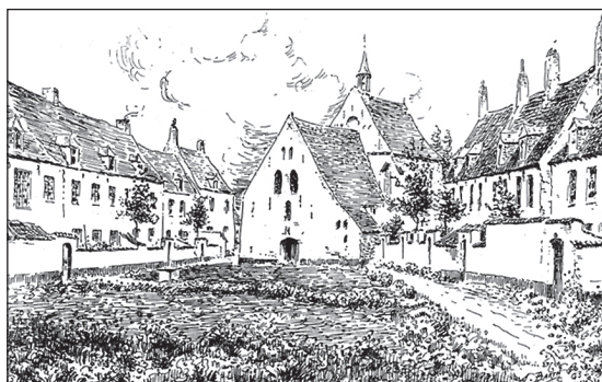
Fig. 4: View of Dixmude beguinage suggested as an example for modern garden city ( L'Habitation à Bon Marché , 1921, n. 1).
