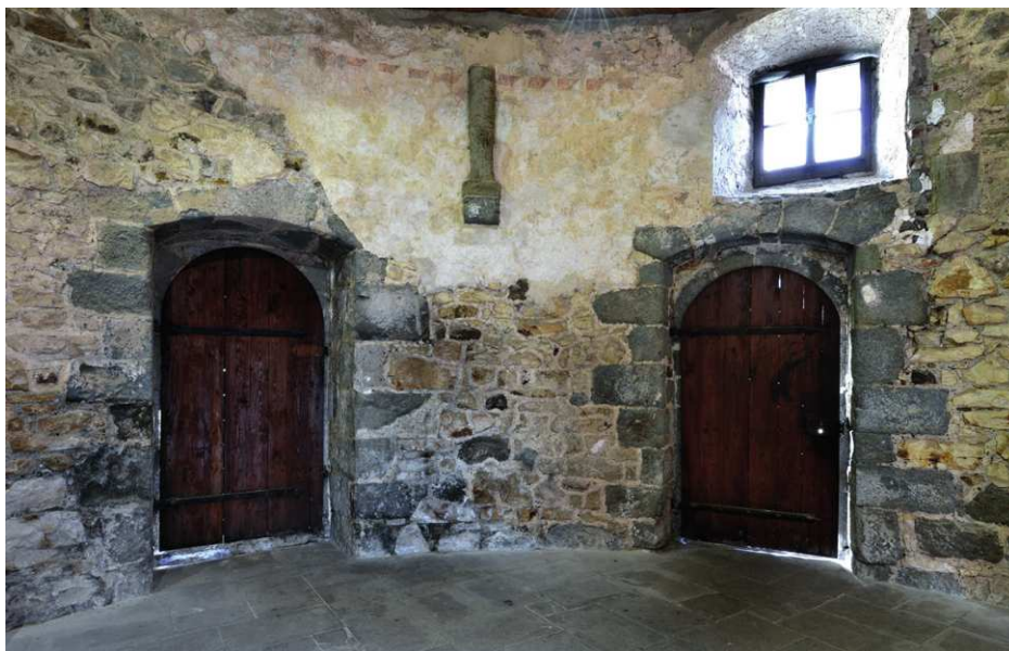
Figure 5: The interior of the Ossuary (St Michael's Chapel) – with Romanesque portals with niches and their straight jambs, built of greyish-green stone blocks. Photo by Lubomír Lužina.
