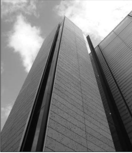
Fig. 5: Recent extension to the British Museum clad in Portland Stone (Photo: William Bondin. ©)
